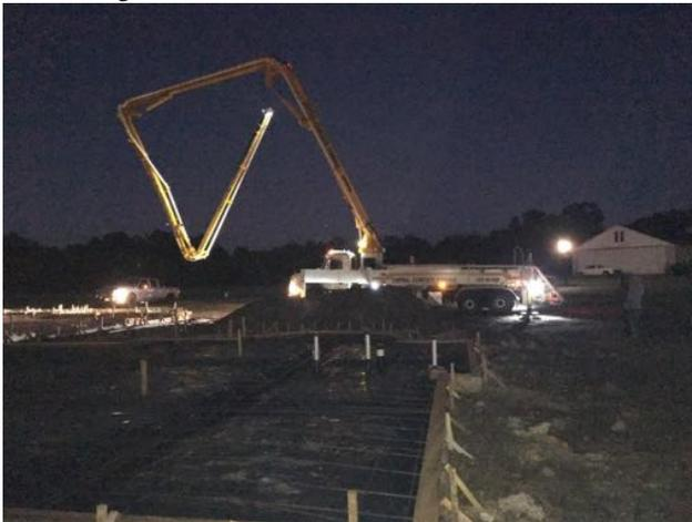
On the appointed day, well before sunrise, the big "Pumper Truck" arrives. This truck has a large boom through which the concrete would be pumped to widespread areas of the foundation. A crew of workers were on hand to spread and smooth the concrete, as well as to set the appropriate shapes for things like slope angles at the hangar and garage.
