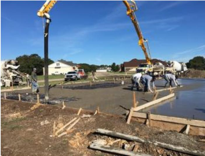
Twenty truckloads of concrete were pumped onto the foundation in about four hours. That's just for the foundation itself, and doesn't include the piers, taxiways or driveways.
